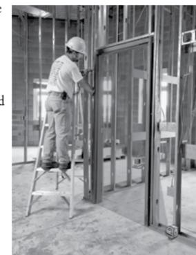
3. Use the Vertical Line Beam to position the floor track.
